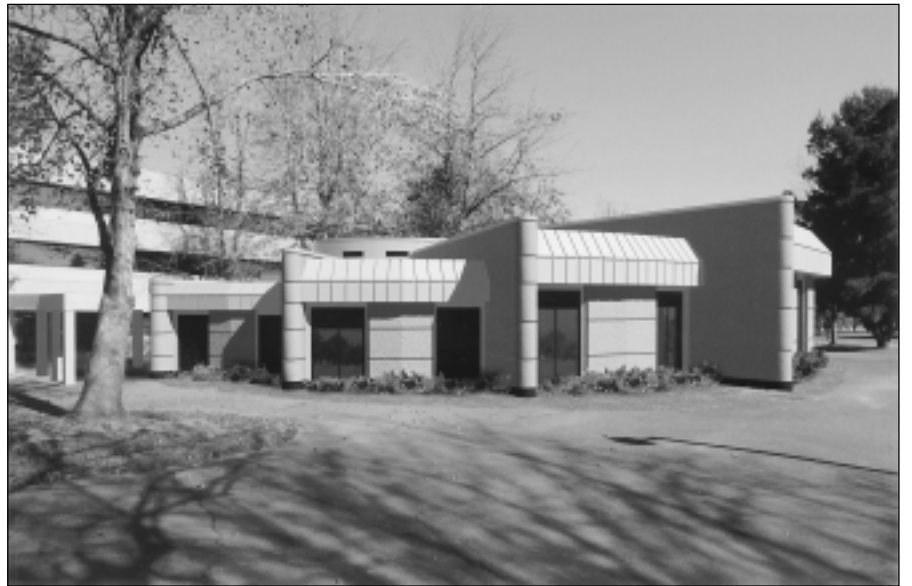
Plans are underway for a 20,000 square foot addition on the south of Tahoe Hall, shown here in an artist's rendering.
