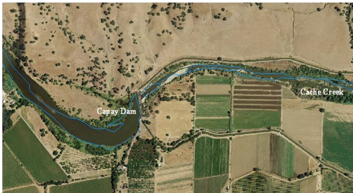
Figure 2.6 Aerial Photograph of Capay Diversion Dam on Cache Creek
