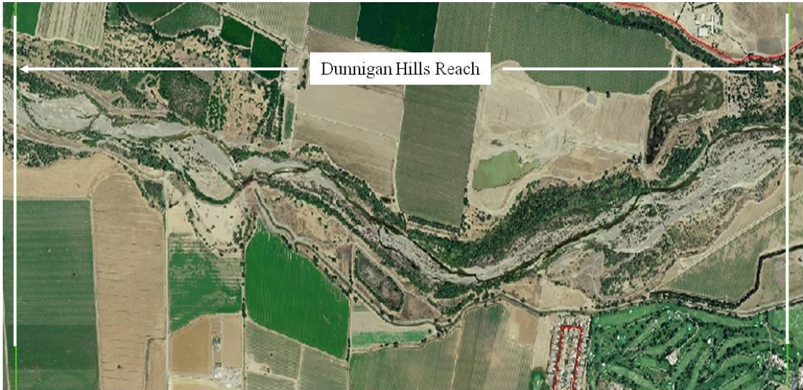
Figure 2.13 Aerial Photograph of Dunnigan Hills Reach
