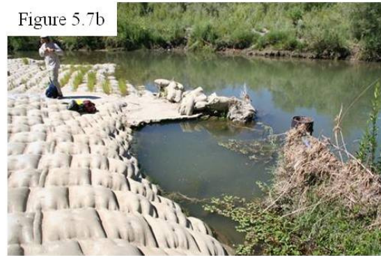
Figure 5.7a-b Photographs of Pacific Palisades Concrete “Pillow” Structure Protecting PG&E Gas Pipeline (Tim Horner, 2008)
