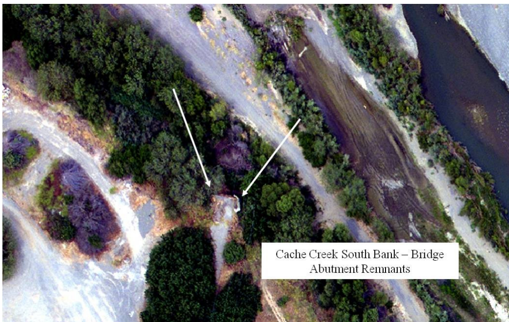
Figure 1.10 Bridge Abutments CR 89 – 2006
