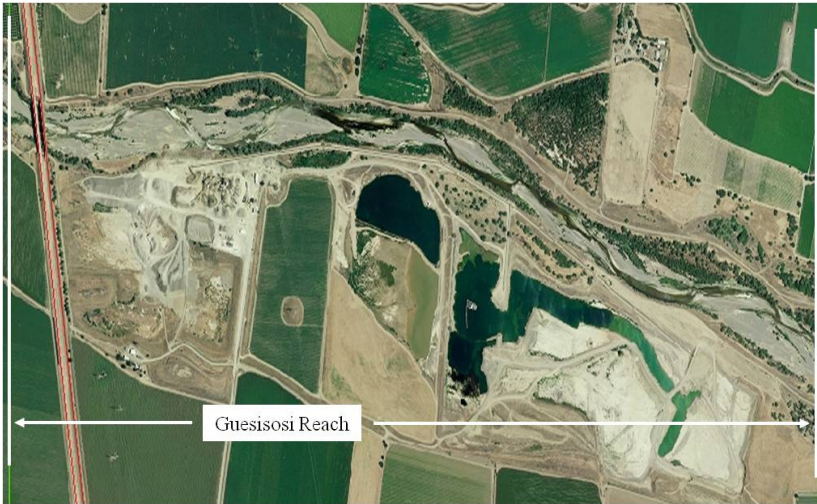
Figure 2.12 Aerial Photograph of Guesisosi Reach
