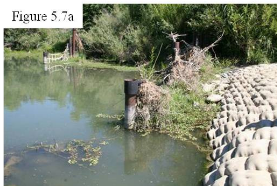
Figure 5.7a-b Photographs of Pacific Palisades Concrete “Pillow” Structure Protecting PG&E Gas Pipeline (Tim Horner, 2008)
