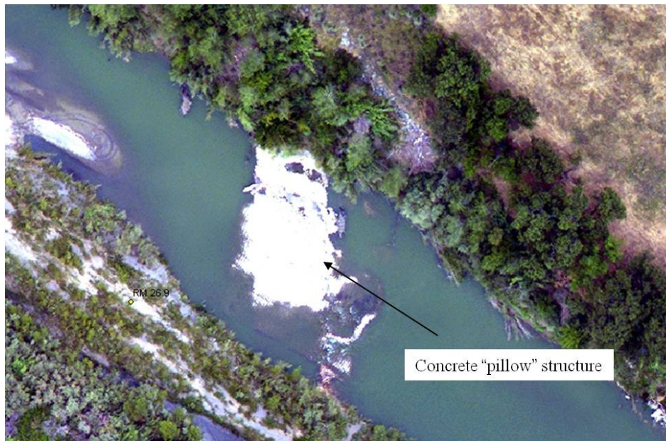
Figure 5.6 Aerial Photograph of Pacific Palisades – Concrete “Pillow” Structure Protecting PG&E Gas Pipeline (2006)
