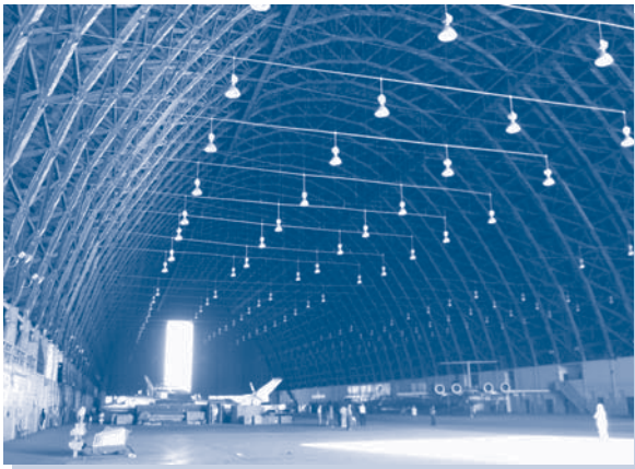
The skeletal interior of Hangar 2
