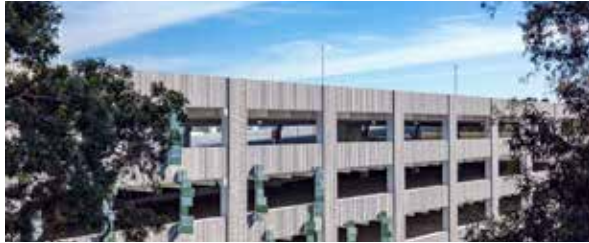
Side view of Parking Structure 5 from Arboretum Way
