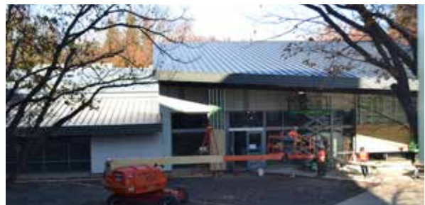
Side view of construction in progress for the new Welcome Center
