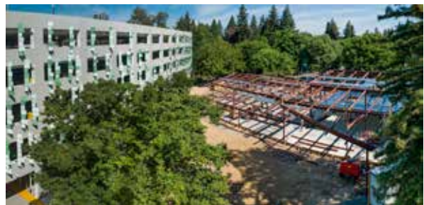
Frame of the Welcome Center next to completed Parking Structure 5
