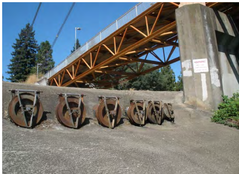
Figure 1 Lift Station #1 Discharge into American River
