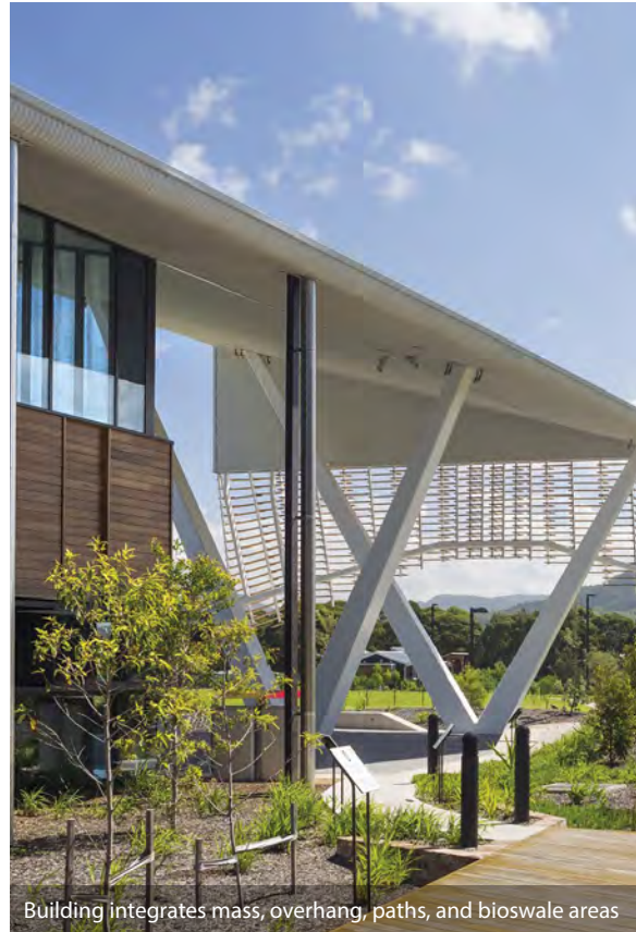
Reduce solar heat gain with exterior sunshade devices
