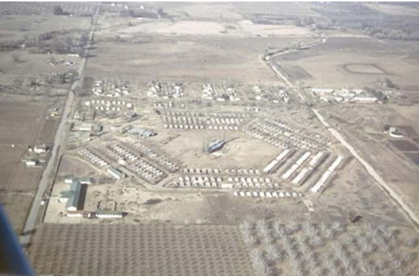
Figure 2. Aerial View of Linnell Camp, 002. Photograph by Unknown, 1939. California Revealed, Tulare County Library, Anne R. Mitchell History Room, Visalia, CA. https://californiarevealed.org
