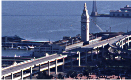
Figure 2. An aerial picture of the double-decker Embarcadero Freeway structure separating downtown San Francisco from the historical Ferry Building and waterfront. Its completion in 1959 marked a turning point in the Freeway Revolt, expanding and radicalizing popular resistance to highway construction. Source: Ferry Building and Embarcadero Freeway , photograph, February 6, 1982.
