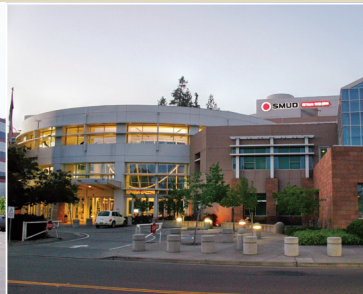
SACRAMENTO MUNICIPAL UTILITY DISTRICT (SMUD)
