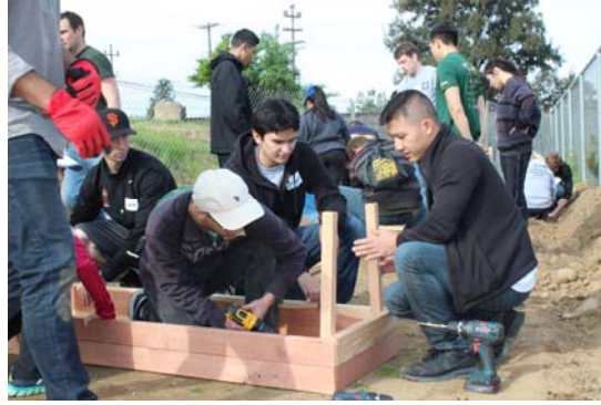
Building the Community Garden planter boxes
