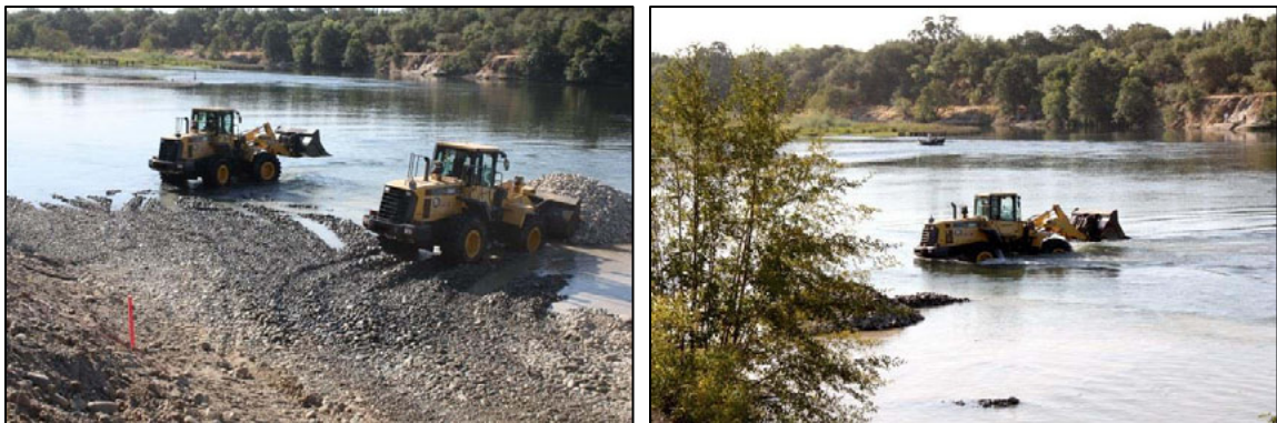
Figure 1.7: Komatsu front-end loaders placing sorted gravel across the Lower Sailor Bar 2012 gravel restoration site in September 2012 (From BOR, 2012)
