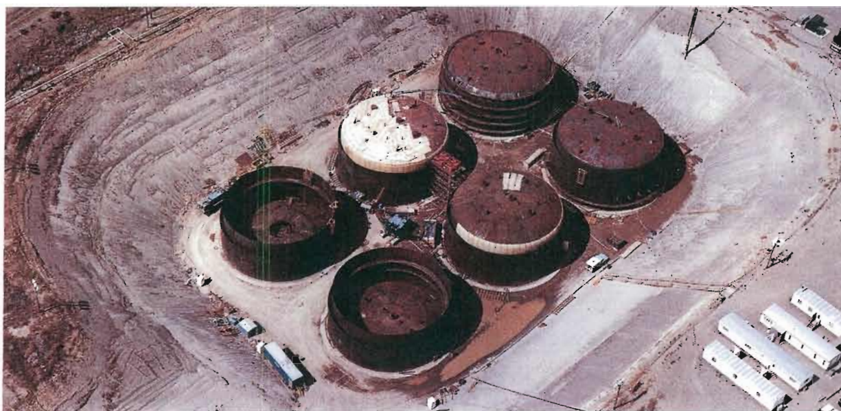
▲ Storage tanks at Hanford, Washington, contain 55 million gallons of high-level nuclear waste. Each tank pictured here holds 1 million gallons.
