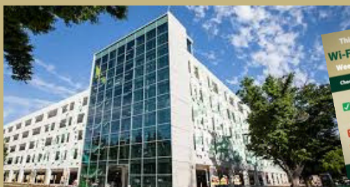
Drive-in Wi-Fi in Parking Structure 5
